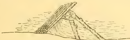
End view of barricade, showing method of construction.
