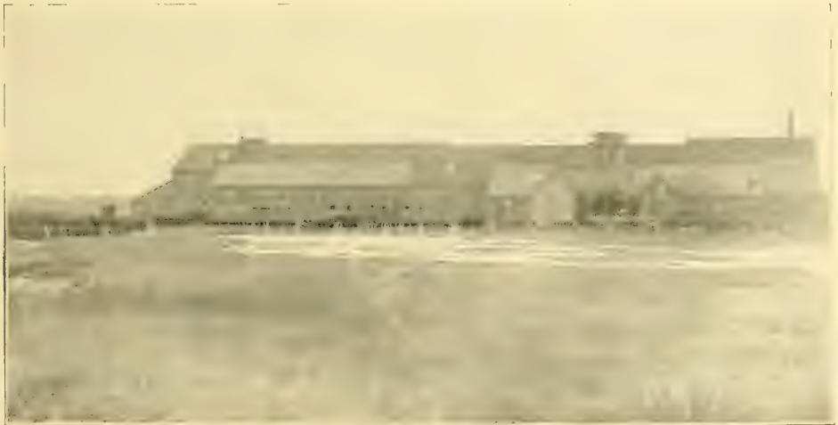
REAR VIEW OF CANNERY AT KUSSILOF, COOK INLET.
