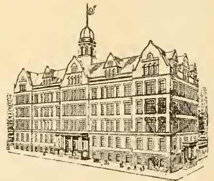
Public School No. 6, Locust Avenue, West Farms
