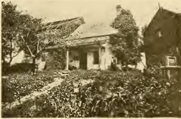
Old Hadley House, Moshulu
