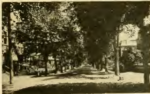
Washington Avenue and 173d Street, Before Widening
