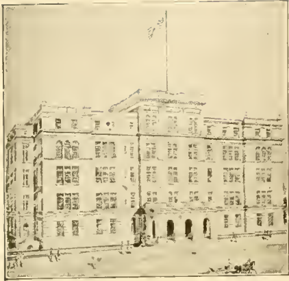
Public School No. 2, Third Ave. near 170th Street
